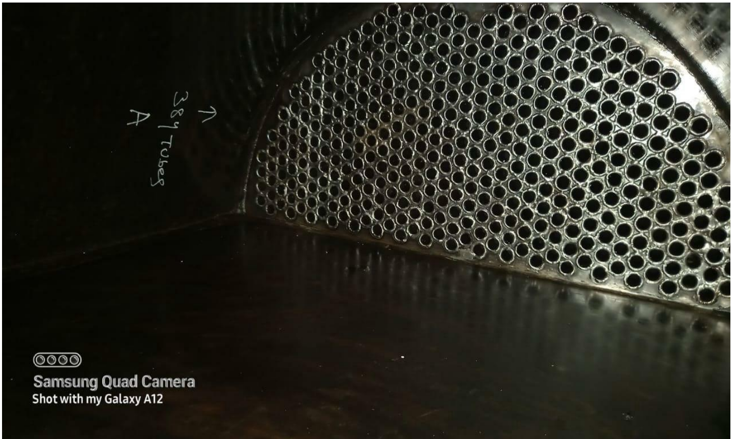
Tube To Tube Sheet Welding
