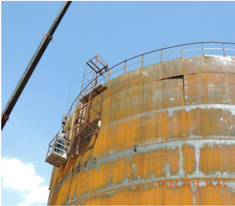
Changing shell plates (inserting)
