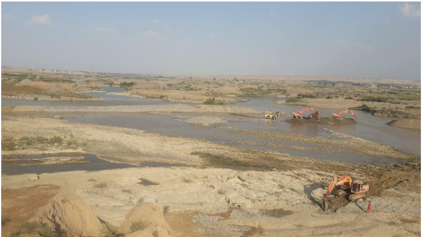
Great Zab River cross open-cut method (Earth work)
